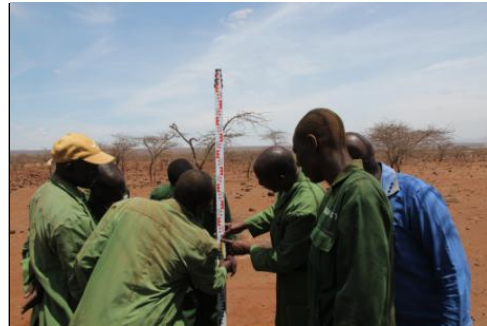
Naga Chief Technology Officer, Sander de Haas, demonstrates proper measurement for the bunds with the MWCT team.
